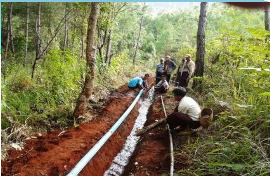
Laying Distribution Pipeline
