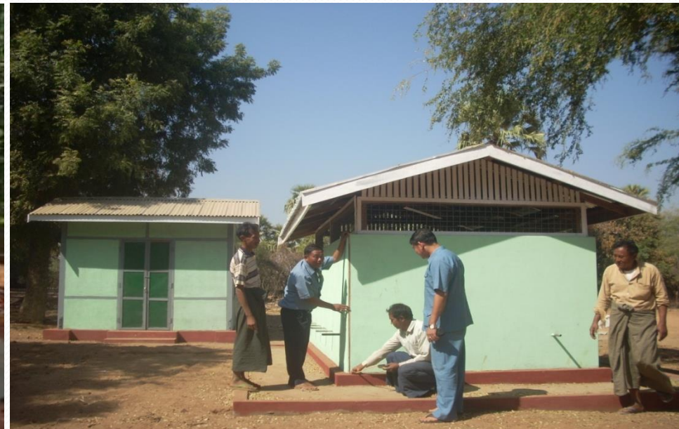
Constructed Tank and Pump House
