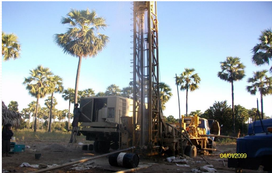
Digging deep tube well
