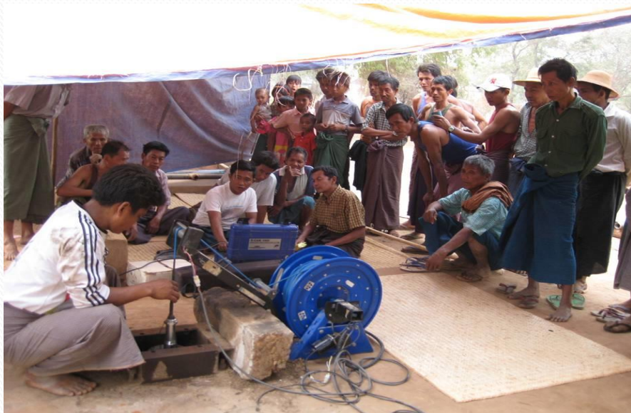
Use of Borehole Camera
